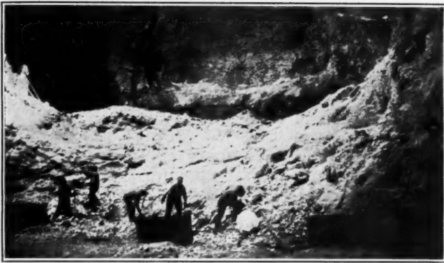
Loading Skips at the Bottom of the Pit
